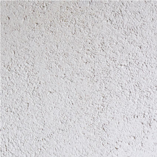
I1. Acoustical Plaster
