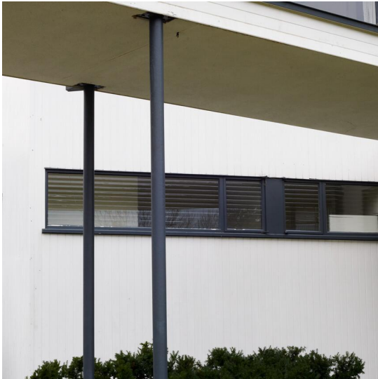
E6. Painted Steel Columns and Casement Windows
