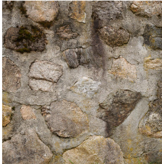
E4. Fieldstone Foundation
