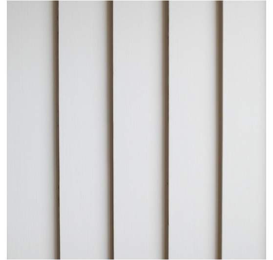
I3. Vertical Interior Clapboard in Foyer
