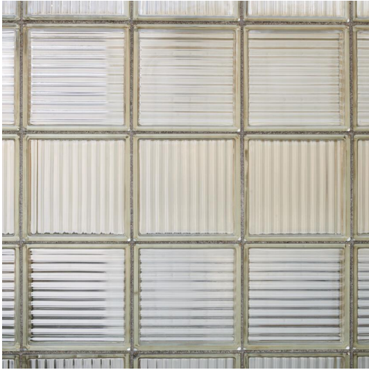
E1. Glass Block Walls – Exterior and Interior
