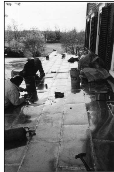
Workers replacing the roof.
