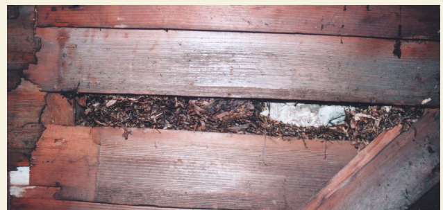
eel grass wall insulation
