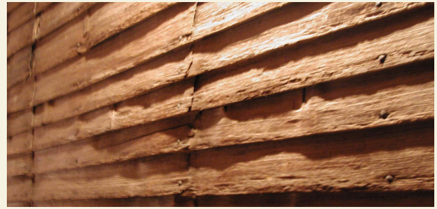
original clapboard siding
