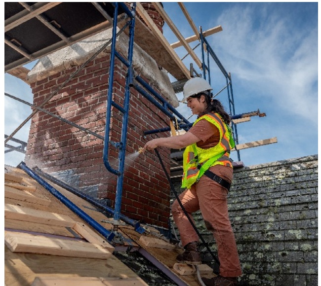
Chimney repair at Beauport, the Sleeper-McCann House, Gloucester, MA
