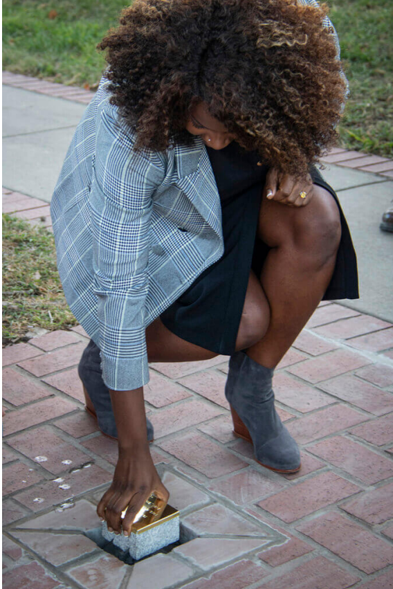
Stopping Stones installation
