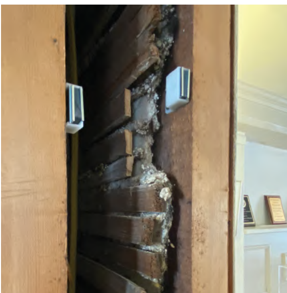
Magnets used to attach the trim while the opening allows a view into the history of the building.
