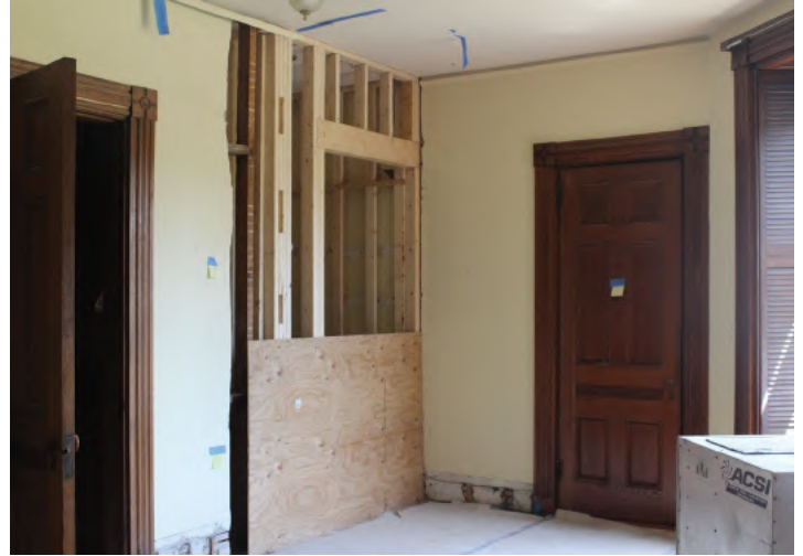
New framing to support the chair lift and its opening.
