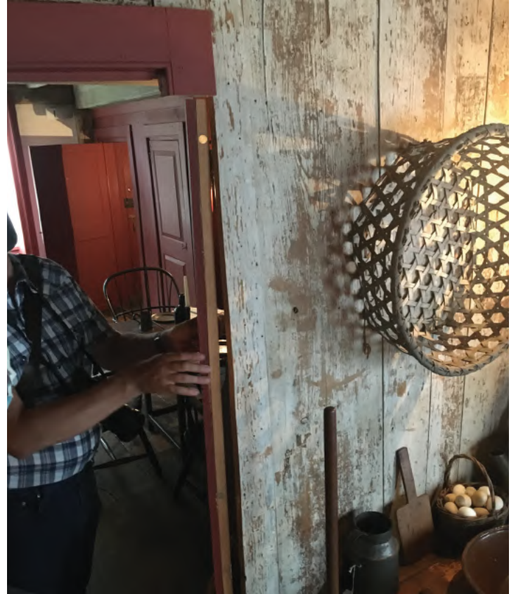
The hinges allow for a section of the board wall to swing open.
