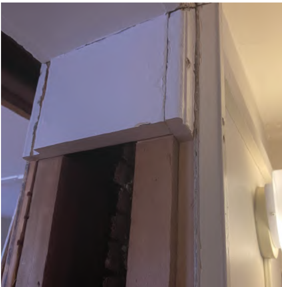
Surgical cuts to remove trim work from the doorway.
