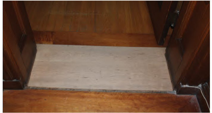
The filler pieces were removed and a new threshold was inserted into the subfloor and flush with the surrounding floor. This image is before staining and final treatments.
