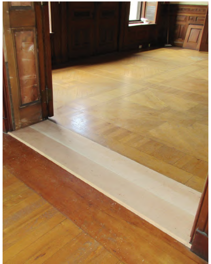
Replacement threshold installed in the same location at ADA compliant levels, before staining and final treatments.
