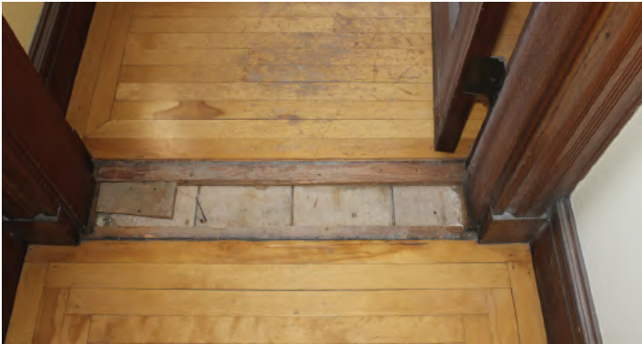
Threshold has been removed, showing the filler pieces used at the Eustis Estate.
