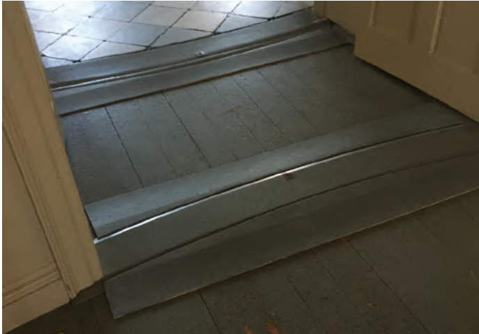
Thresholds and wooden threshold transitions at the Gore Estate.
