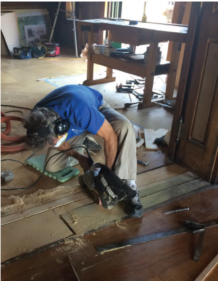
Historic New England preservation carpenter sanding the existing filler pieces once the threshold was removed.
