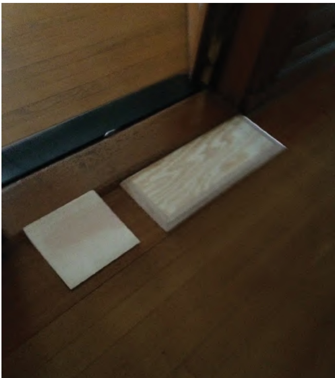
Mock-ups at the Eustis Estate to review a rubber transition strip, as well as two variants of wood.
